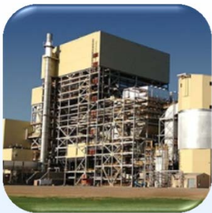
Utility Steam Generation
